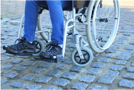
The cobbles used to supposedly control vehicle speed can trap the front wheel of a wheelchair, causing it to tip over
