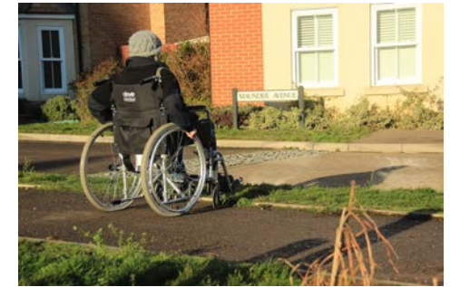
Obvious crossing points are missing wheelchair ramps.
